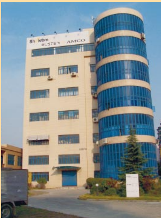
Fig. 2: Production building at Shui Dian Road in Shanghai
