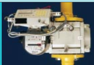
Fig. 5: Vertical installation of RVG with S1D index and EK-88/K volume corrector
