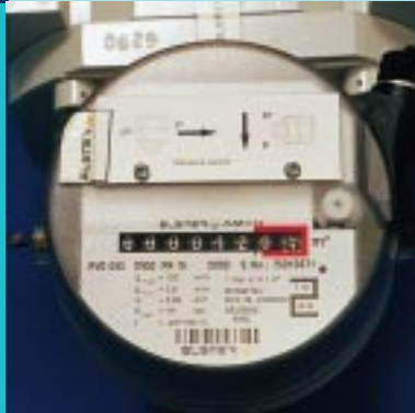
Fig. 2: Upper index hidden. Flow directions shown on the cover plate.
