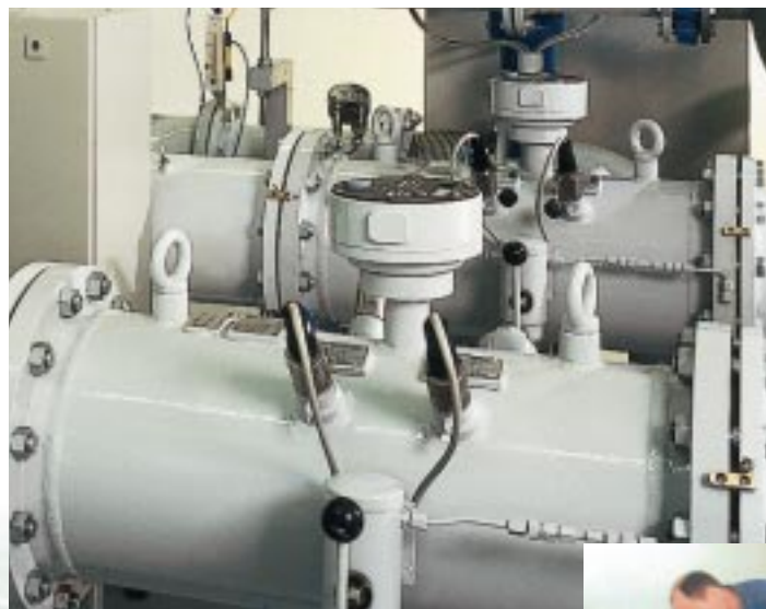
Turbine gas meters, measuring range from 160 m 3 /h up to 1600 m 3 /h
