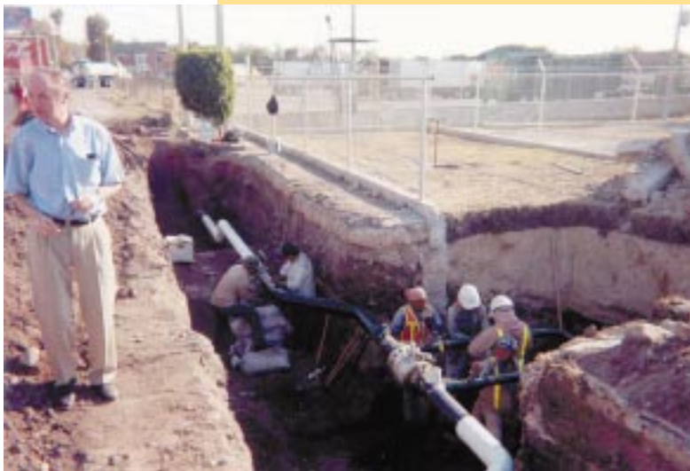
Preparing to install a new station in Queretaro
