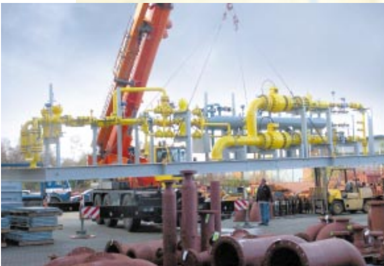
The Douglas skid ready to be installed in the kiosk
