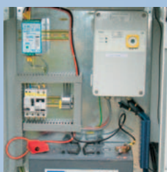
Fig. 3: The FE260 with power supply and backup battery
