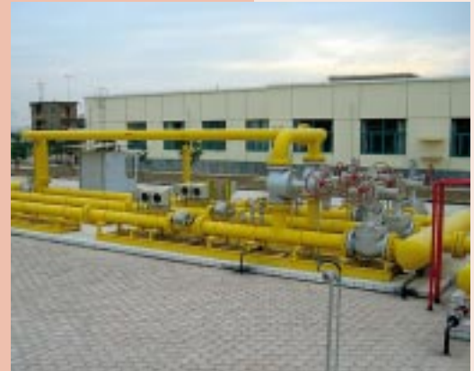
Fig. 2: Hengmen Power Plant station
