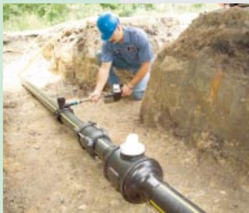
Fast, safe and easy installation of a service line onto a main with Perfection's complete polyethylene mechanical system
