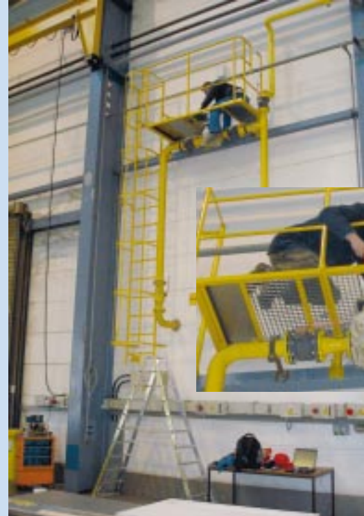
Fig. 1: EK260 – Installation on a pipeline bridge
