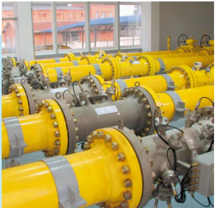
Fig. 4: Ultrasonic master meters lined up in the Secondary Standard
