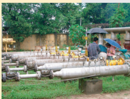
Fig. 2: Natural gas station outside Dhaka
