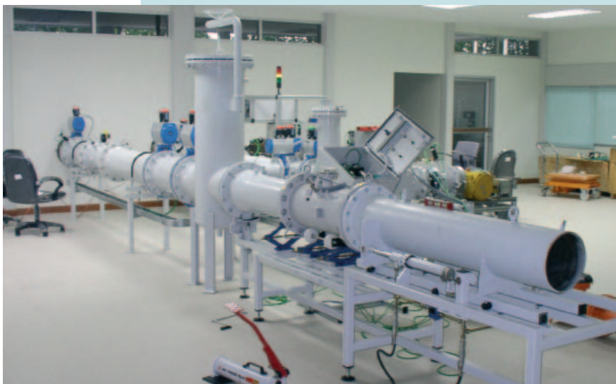
Installation at the customer's premises
