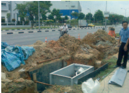
Orpheus 4 module being installed underneath a footway
