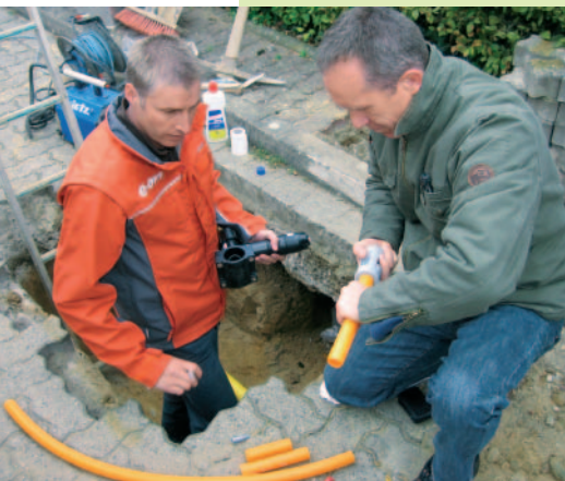
Torsten Lotze (E.ON Avacon) and Torsten Hain (HTI Collin) when mounting Permasert® couplings
