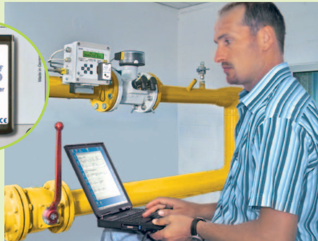
Fig. 1: Wireless connection to laptop using Bluetooth LIS-200 adapter on EK260
