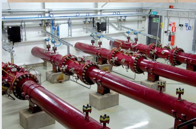
16" metering lines with Q.Sonic-5S meters
