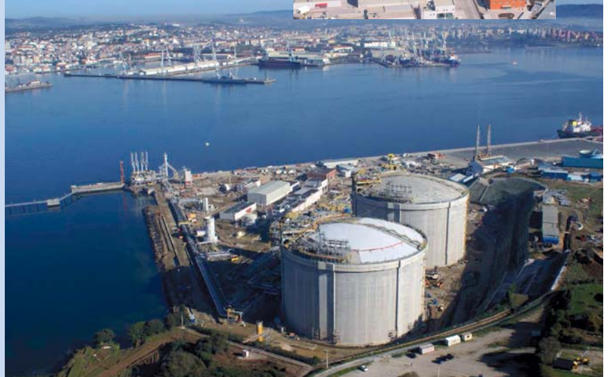
Reganosa LNG terminal on only 9 ha with the two eye-catching 150,000 m 3 full containment LNG storage tanks
