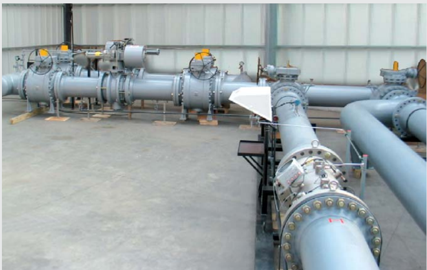
Outlet section, ultrasonic meters and flow control valve outlet section during factory inspection
