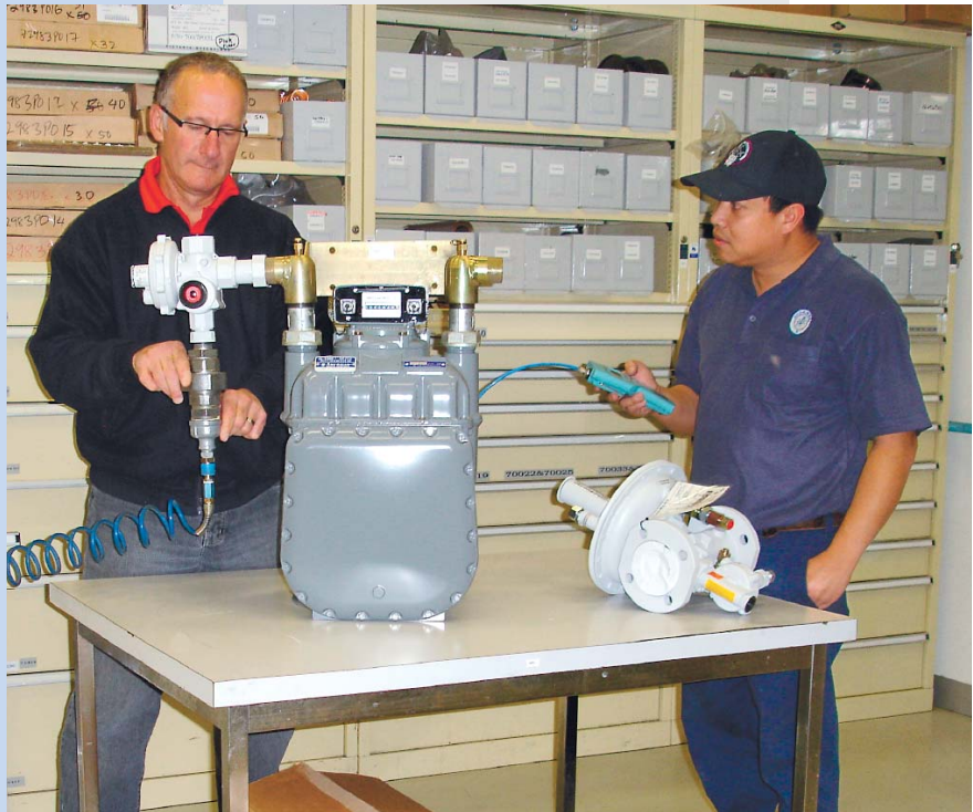
Noel Critch and Max Prado are testing the M2R 75/AL 1000 installation
