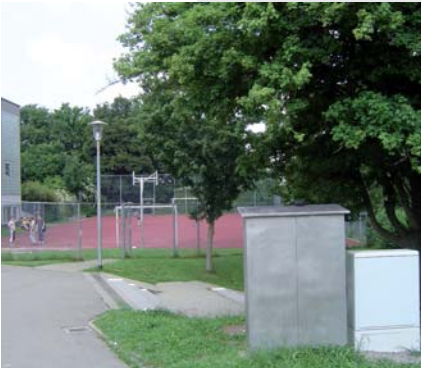
Fig. 1: Gas station in direct proximity to a street lamp
