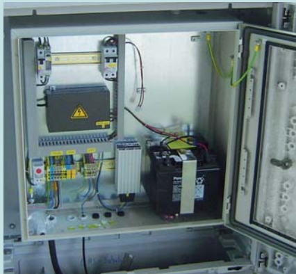
Fig. 2 and 3: Separate control cabinet with rechargeable battery, charge controller and freeze protector for the energy supply of modem and volume corrector
