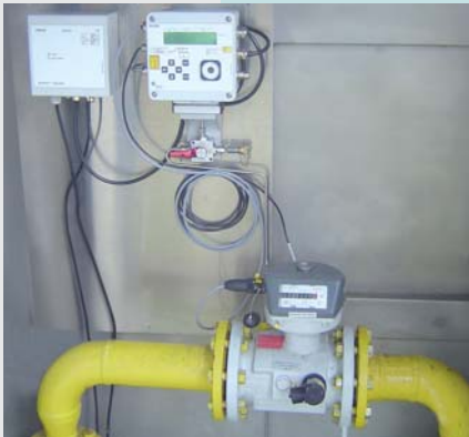
Fig. 2 and 3: Separate control cabinet with rechargeable battery, charge controller and freeze protector for the energy supply of modem and volume corrector
