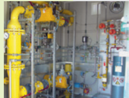
Fig. 5: Volumetric metering system and LPG conditioning system
