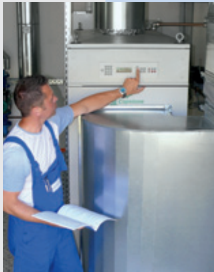
Micro gas turbine in a gas regulating and metering station
